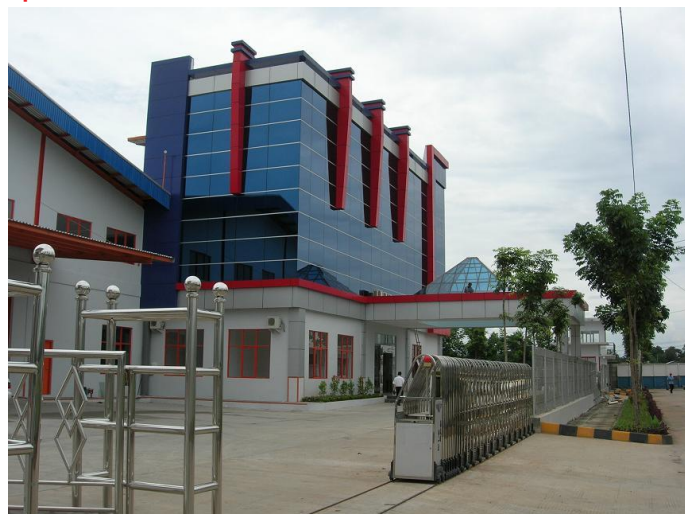
Figure 5: Tokyo Radiator JV is on track for Apr 13 initial operations
